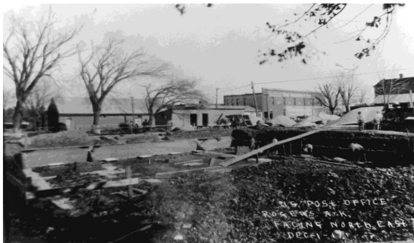
Beginning construction of Post Office, 1917, looking NE, Courtesy Rogers Historical Museum
