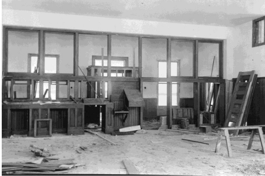
Construction of craftsman style clerks' windows, back of building, south side, 1918 Courtesy Rogers Historical Museum
