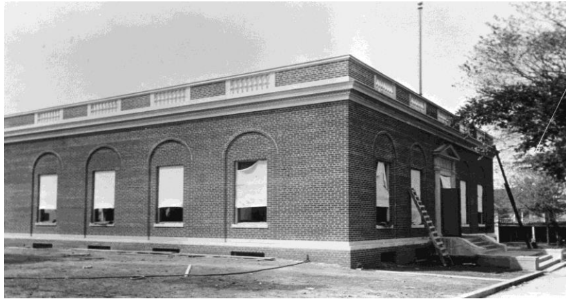
Post Office construction, 1918, view of east side, Courtesy of Rogers Historical Museum
