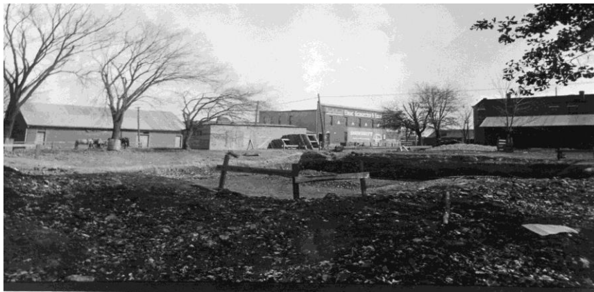
Beginning excavations on Post Office, looking NE, 1917, Courtesy Rogers Historical Museum
