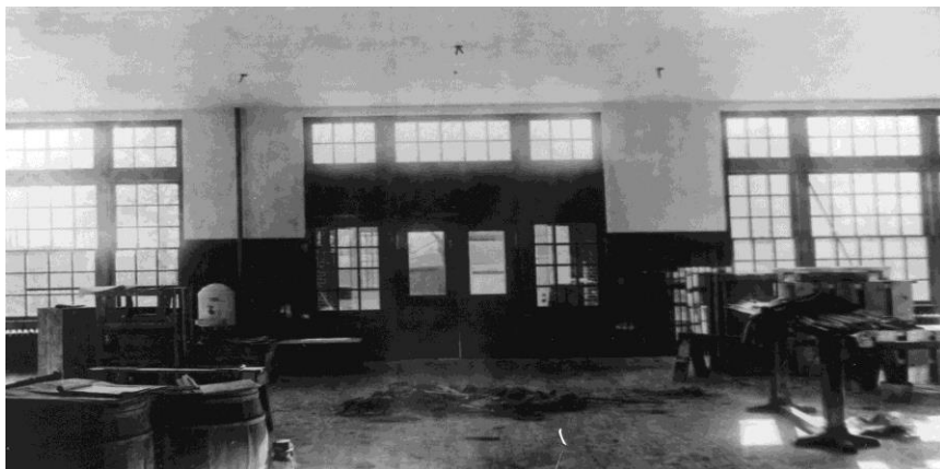
Construction of Interior, front, facing north, 1918, Courtesy Rogers Historical Museum
